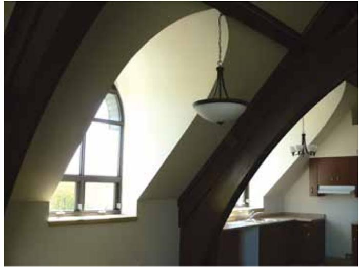
*The adaptive reuse of St. Thomas Church in Waterdown, ON required a new second floor inserted at the upper level of the original nave. The firm maintained the original wood arches and refurbished the original light fixtures.*
